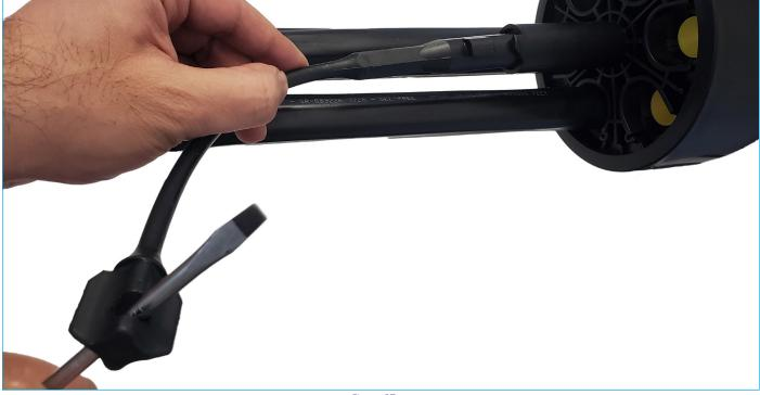
10.9 Place a large tie wrap or vinyl tape around all the cables just beyond the end of the tail.
