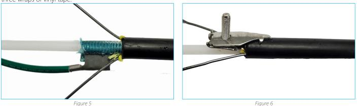
8.4 If using shield bond connector, push the lower plate of the bond clamp under the inner shield so that the stud bolt is positioned between strength members. Place the upper plate of the B-Bond clamp over cable jacket. See Figure 6.
