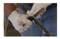
Apply Electrical Tape to Protect Breakout
