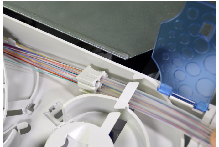
6.1.8. Open the lids. Push / slide all transportation tubes one by one into the tray.
