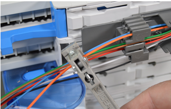
6.1.2. Strip the loose tubes at the marked point and clean the fibers.
