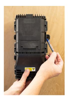
2.1 Mark the four (4) positions for the screws in the wall (mounting tabs).
