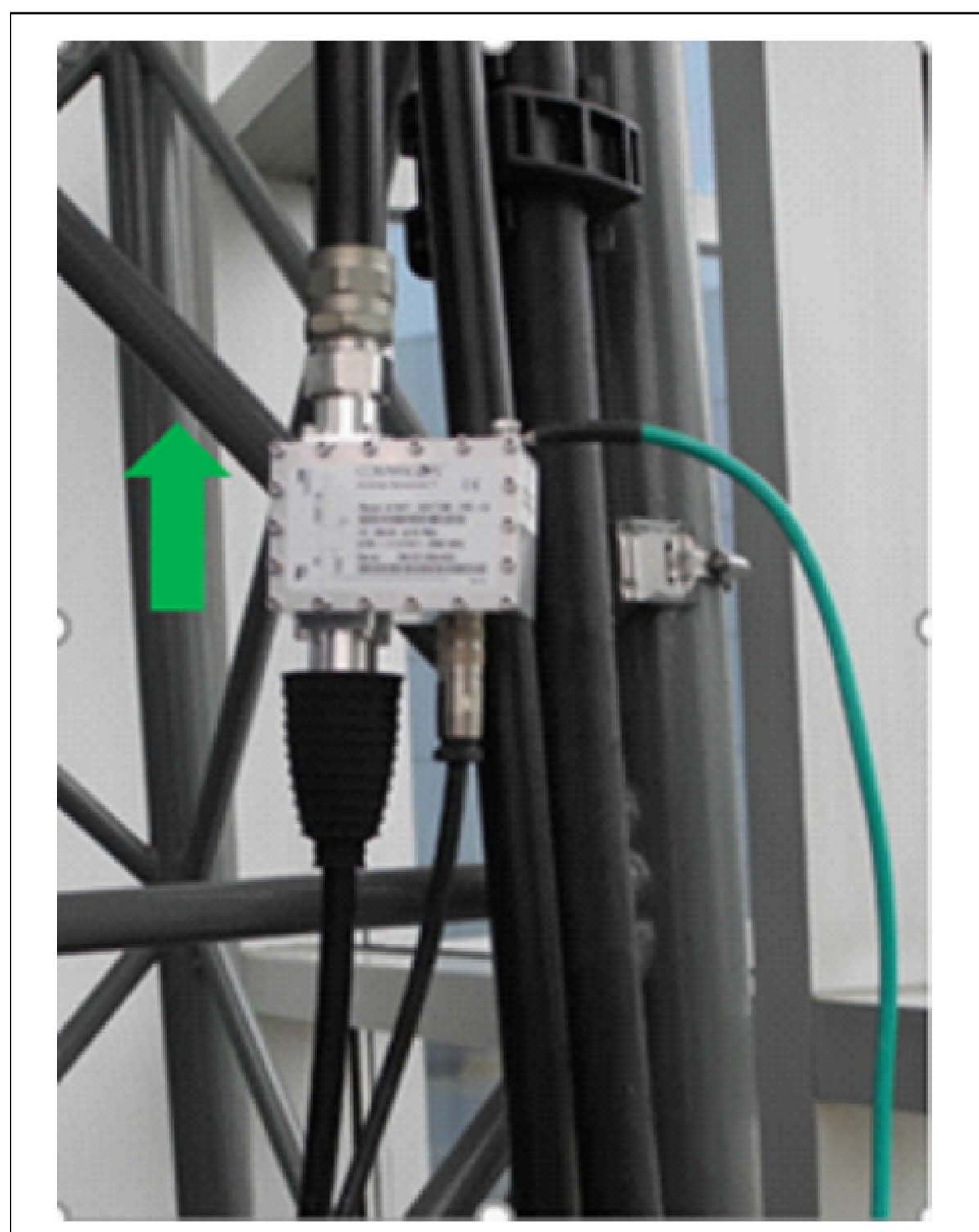
Figure 3. Recommended vertical position
