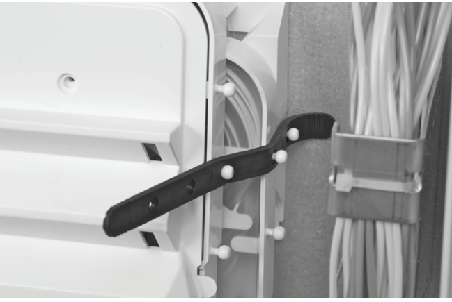
6.4 Secure the patch trays with the rubber flex part, as shown.
