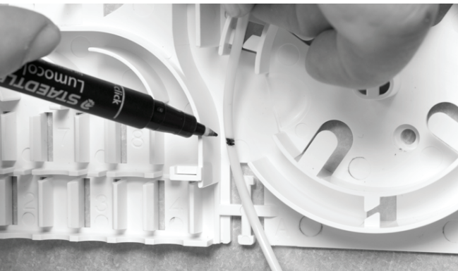
2.4 Route the loose tubes to the base tray. Mark left and right side of the loose tube at their position on the base tray.
