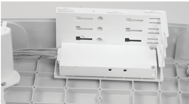
4.2 Install the splitter into the holder and route the pigtails via the bend control.
