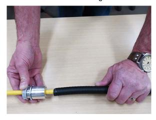
8. Thread the armor fitting onto the base of the cable armor. Tighten until snug.
