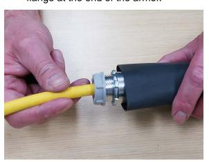
Using the most effective distance and lowest effective heat setting on the heat gun, shrink the heat shrink tube until it is fully compressed.
