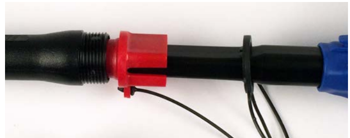
Cleaning Tool Pushed into HMFOC Pinned Connector
