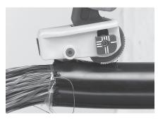
**4a.** In order to install the shield continuity wire, cut the cable jacket over a length of 20 mm and a width of 10 mm.
