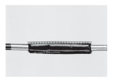
**23.** After installation allow the block to cool to ambient temperature before moving the cable. **Pressurise the cable after 24 hours.**
