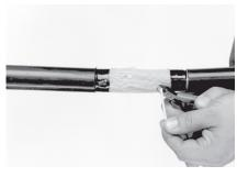
**6.** Insert the channelling pins through the conductors at 10 mm from each other. Insert completely and cut-off the excess. Use the left over pieces until the pin is totally used up. Do not force the channelling pin.
