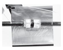
**12.** Centre the sleeve over the adhesive bags and mark the sleeve ends on the cable.
