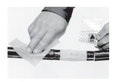
**8.** Remove the cleaning tissue from its packaging and clean the cable jacket on both sides of the cable opening over a distance of 100 mm.
