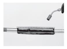
**22.** After complete installation of the second sleeve give a post heating of 1.5 seconds around the middle of the sleeve.
