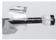
**13.** Wrap the aluminium cable protection foil around the cable, the blue line matching the marks on the cable jacket. Smooth the aluminium foil with a blunt tool.
