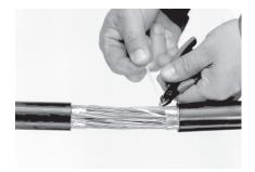
**3.** Remove all unit tapes in the cable opening. Spread the conductors evenly so that there are no groups of conductors tightly bundled. The conductor bundle diameter should be about 5 mm to 10 mm larger than the original cable core diameter.
