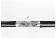
2. Remove the jacket over a distance of 120 mm. Remove the cable wraps but leave 10 mm on each side of the cable opening.
