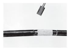
10. Flame brush the cleaned and abraded cable jacket for 10 sec. Point the flame away from the cable opening. Make sure that the entire cable surface is touched by the flame.
