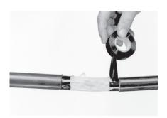
**5.** Wrap the mesh around the cable opening and secure the mesh on both ends of the cable opening with PVC-tape.
