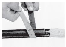
**9.** Abrade the cable circumferentially over the cleaned distance.
