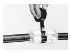
**11.** Wrap the adhesive bags around the cable opening, mesh side down. Secure in the middle with PVC-tape.
