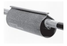
**19.** Immediately align and wrap the second sleeve over the installed and post heated sleeve. Position the channel opposite to the first channel (180°).
