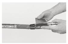
12 Apply the adhesive strip, starting under the grounding wire and ending over the wire.
