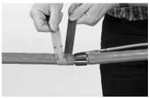
8 Abrade the cable jacket circumferentially over a distance of 10 cm at both sides of the roll spring.
