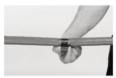
4 Place 1 wrap of the roll spring over the copper mesh.
