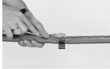
5 Strip the grounding wire over a length of 14 cm. Spread the wires and place them on the roll spring.
