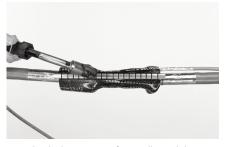
15 Shrink sleeve circumferentially until the temperature sensitive paint has changed from green to black.
