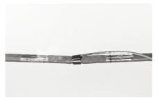
11 Flame brush the cable jacket between the aluminium tapes for about 10 seconds. Make sure to treat the entire jacket surface with flame
