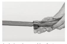
6 Apply another wrap of the roll spring. Bend the grounding wire to the other side.
