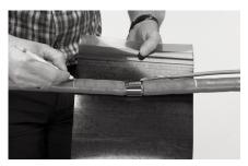
9 Center the sleeve and mark the sleeve ends on the cable.
