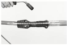
16 Shrink gradually and progressively the sleeve to one end moving the flame circumferentially around the closure. Return to the starting point at centre and repeat for the other half.
