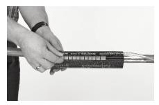
13 Position the sleeve. Pull stainless steel channel over the rails.
