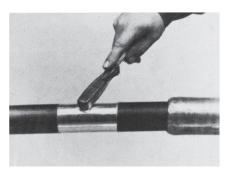
**7** Dress the aluminium cable tape with a blunt tool to smooth sharp edges.
