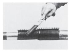
**13** Press the chanel with a blunt tool to follow the transition from lead to cable.
