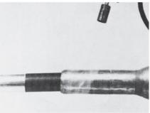
**9** Preheat the lead surface over abraded length up to  $\pm$  60°C (hot to the touch).
