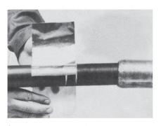
**6** Apply aluminium cable tape on the cable jacket away from the lead starting from the inner mark.
