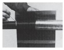
**4** Centre the wraparound sleeve, half over lead, half over the cable and mark the end of the sleeve on cable jacket.
