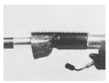
**12** Continue shrinking the other half of the sleeve on the cables moving circumferentially towards the end of the sleeve.
