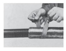
**3** Abrade circumferentially the lead surface over a length of  $\pm$  20 cm.
