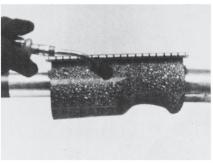
11 Recover the sleeve starting from the centre moving circumferentially (360°C) towards the lead part. When the paint has completely changed to black progressively move towards the lead part.
