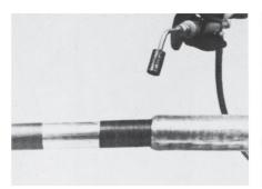
**8** Flame brush the cable area between lead and aluminium tape for about 10 seconds.
