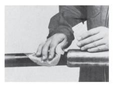
1 Remove solvent impregnated tissue from its package and clean the cable jacket for a distance of  $\pm$  20 cm.
