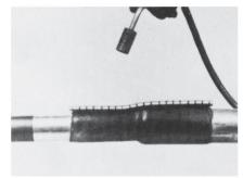
14 Apply additional heat along the entire channel area for at least 20 seconds to ensure good flow of adhesive. Adhesive must flow from the ends of a sleeve properly shrunk.
