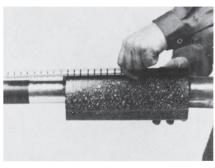
10 Wrap the heat-shrinkable sleeve around lead and cable. Pull the steel channel over the rail. The channel must protrude the same distance at each end. Centre the sleeve versus the lead/cable jacket-transition.
