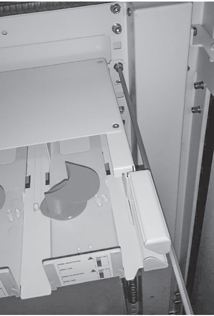
5.2 Hold shelf in place and install first onto one side of the cabinet.
