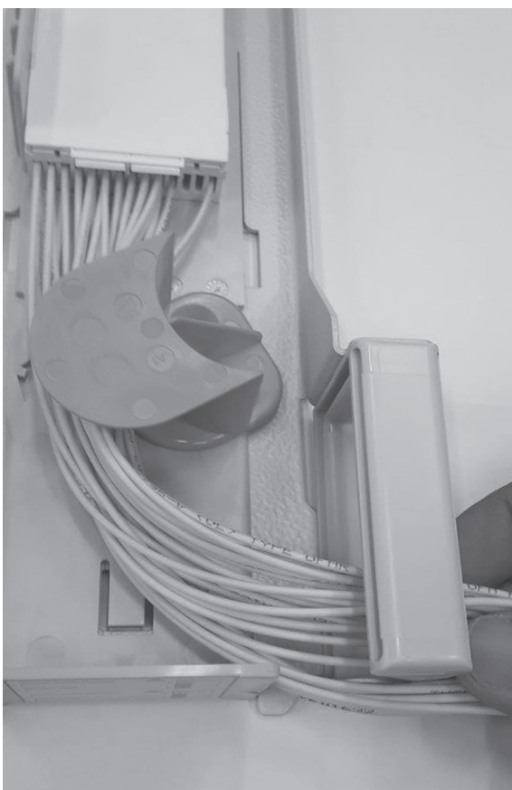
6.3 Guide the patchcords besides the radius limiter and through the cable ring.
