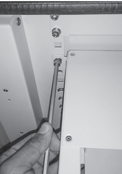
5.3 Hold shelf in place and install onto the other side of the cabinet.
