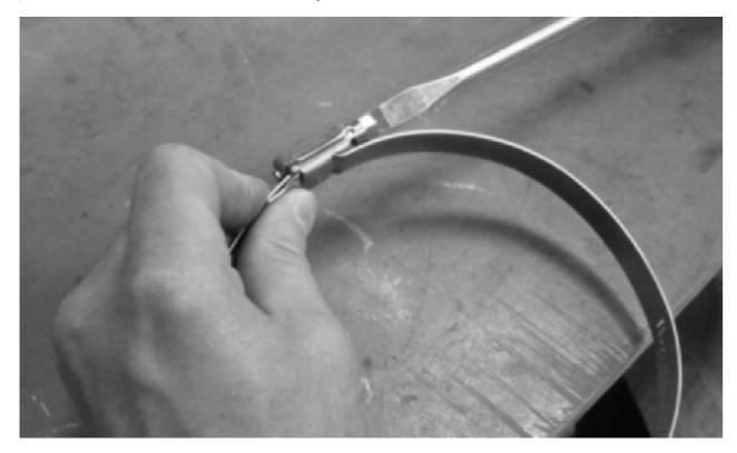
3) Insert the clamp into mounting holes.
