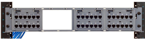
Figure 10 Reinstalling the Module
