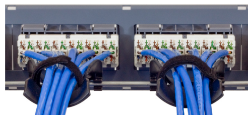
Figure 13 Routing and Retaining the Cables
