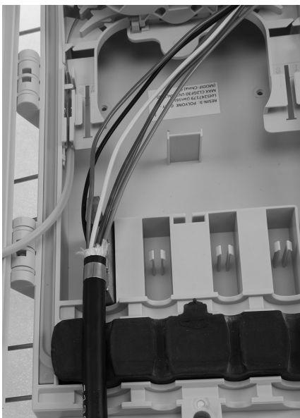
1. Install feeder cable (L or R side)
